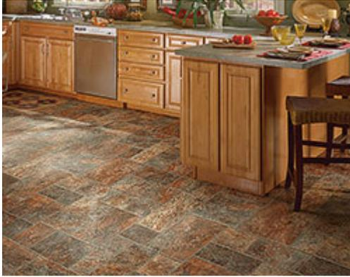
With **printed vinyl**, patterns are printed using a paper top coat placed directly on a thin vinyl surface and then covered with several layers of clear vinyl or urethane to produce a protective wear layer. Also referred to as rotovinyl, this type of vinyl is a more affordable option to inlaid vinyl but is less durable.
